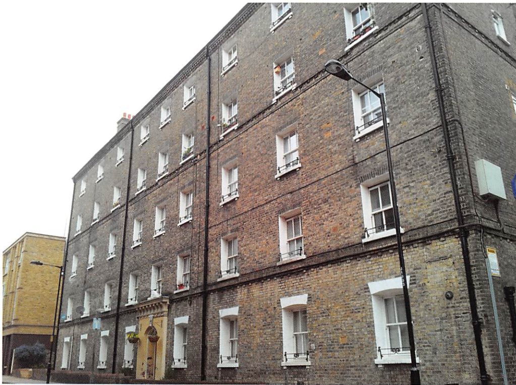
▲ Source E A picture showing Peabody buildings in Whitechapel in 2012.
